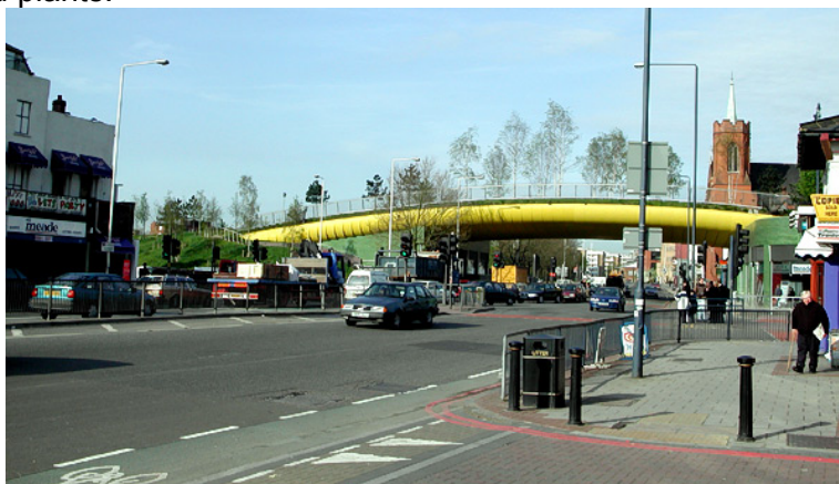
The Green Bridge
